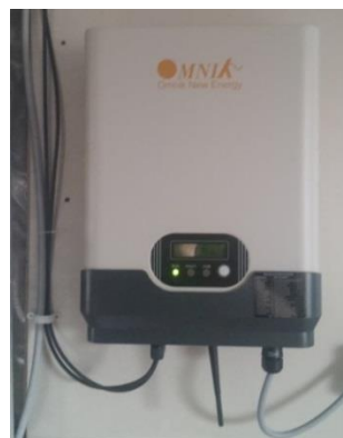
Figure 4. Small wall mounted photovoltaic inverter (1,75 kWp) indoor on an attic.
