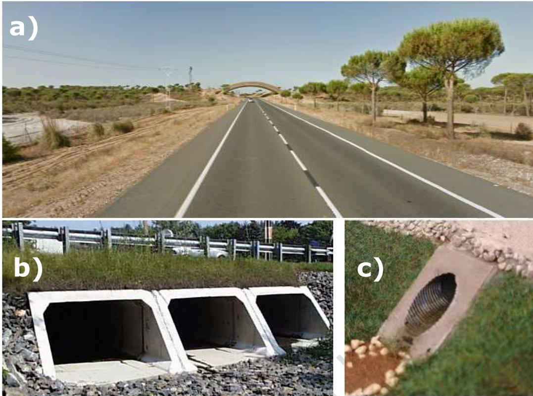
**Figure 3.51: a) example of a bridge crossing as a migration pathway for large endangered animal species b) a typical box type road culverts for drainage conveyance and c) a typical grooved pipe road culvert.**
