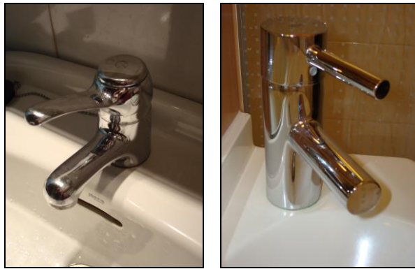
Figure 5: Examples for single lever monobloc (single-hole) mixer taps Source: A. Uihlein
